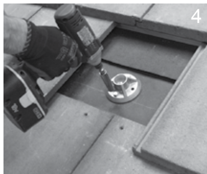
Align Q Base over rafter center and drill 2 each 7/32" pilot holes. Place grade 8 Machine Bolt under Q Base in hex slot, threads pointing up. Lag Q Base into Rafter on Marks.
