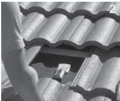
Locate center of rafter and Mark with a felt pen.
