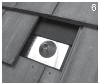
Take care to do a quality installation – when using the paper method, cut a piece of paper 18" wide to slide under the course above, and over the Primary Flashing of the Mount.
