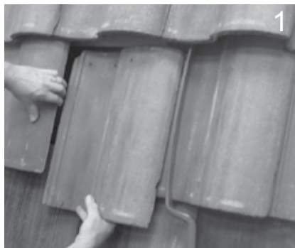
Remove Tile at selected location of Mount.
