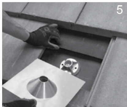
Carefully clean the building paper then install Primary Flashing in either a three course method, or properly lapped paper method. Now is a good time to apply sealant to the flashing opening.
