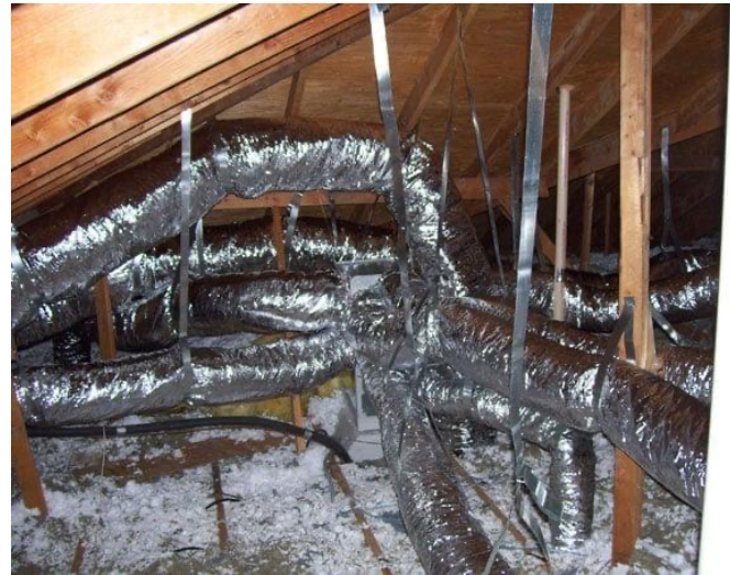
Typical Higher Duct Static
